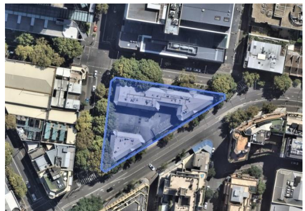
Figure 7: aerial, 37-69 Union Street
